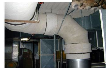
ASBESTOS CEMENT LAB FUME HOOD EXHAUST DUCT
