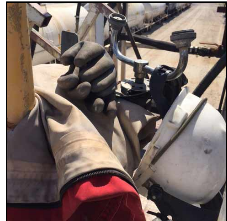
Figure 1.3 Obstructed eyewash station
