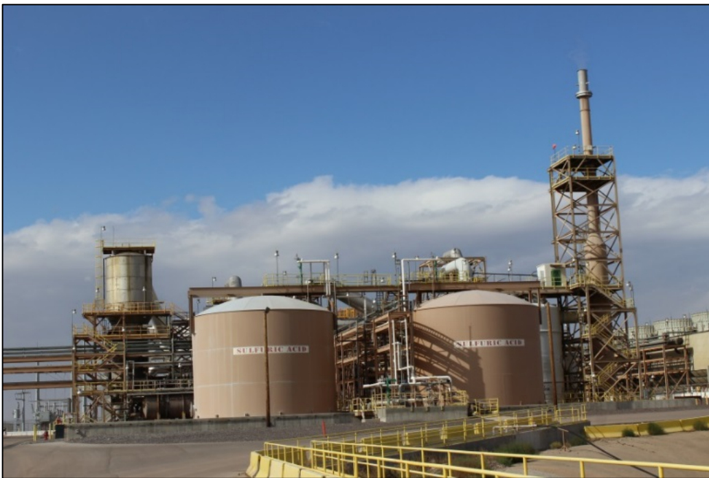
Fig. 17 Potential for vapors, gases, and fumes at sulfuric acid plants
