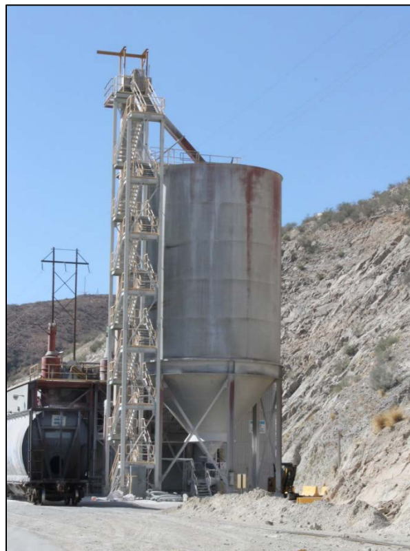
Fig 22 Silos have inwardly converging walls
