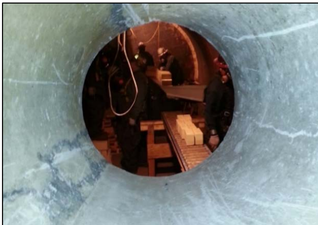
Fig. 1 Rebricking in a confined space
