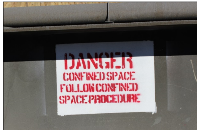
Fig. 36 Confined space signage
