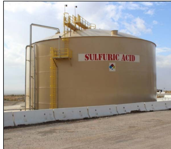
Fig. 6 Acid tank is a hazardous atmosphere
