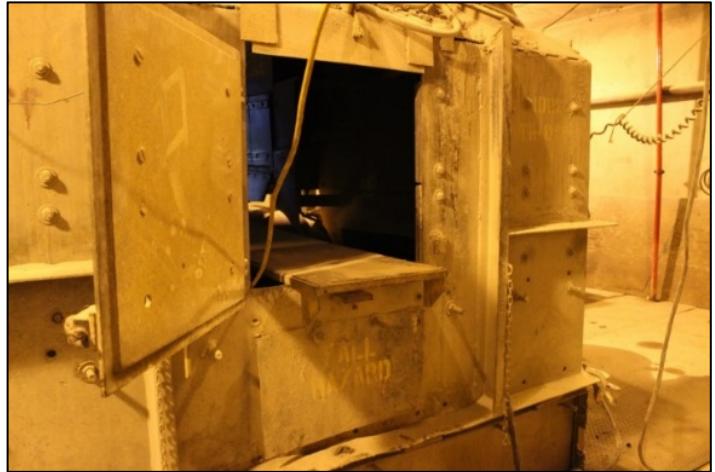
Fig. 3 A crusher chute is large enough to enter
