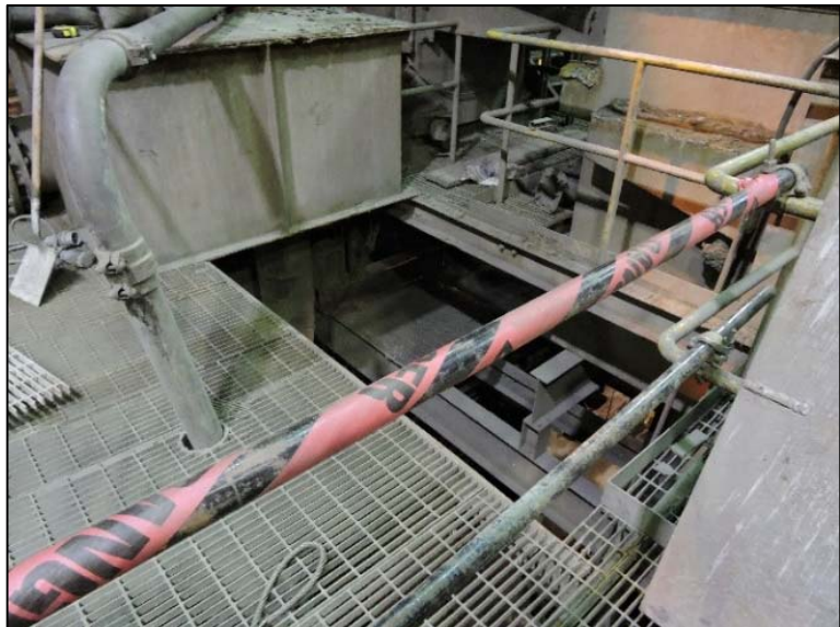
Fig. 35 Even when guarded, open holes pose a risk
