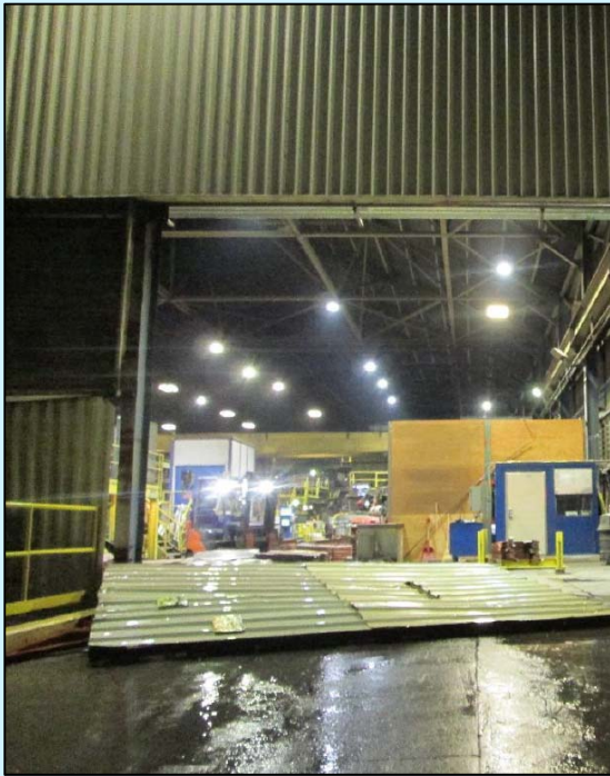
Fig. 5 Door that fell
