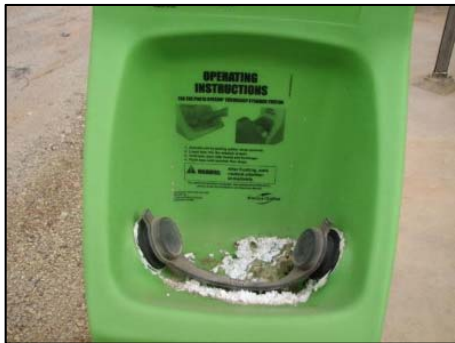
Fig. 29 Eyewash station with build-up
