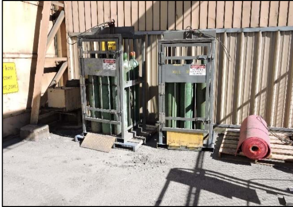
Fig. 17 Properly stored tanks
