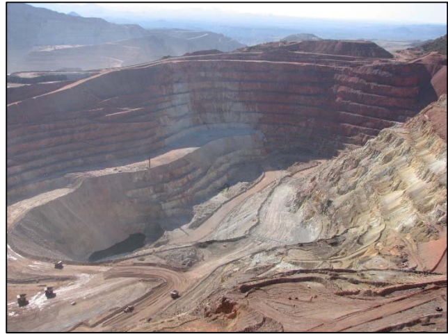
Fig. 37 Visible highwalls and benches
