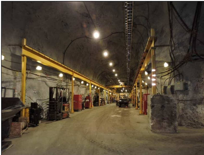
Existing Hazard(s) / Potential Consequence
