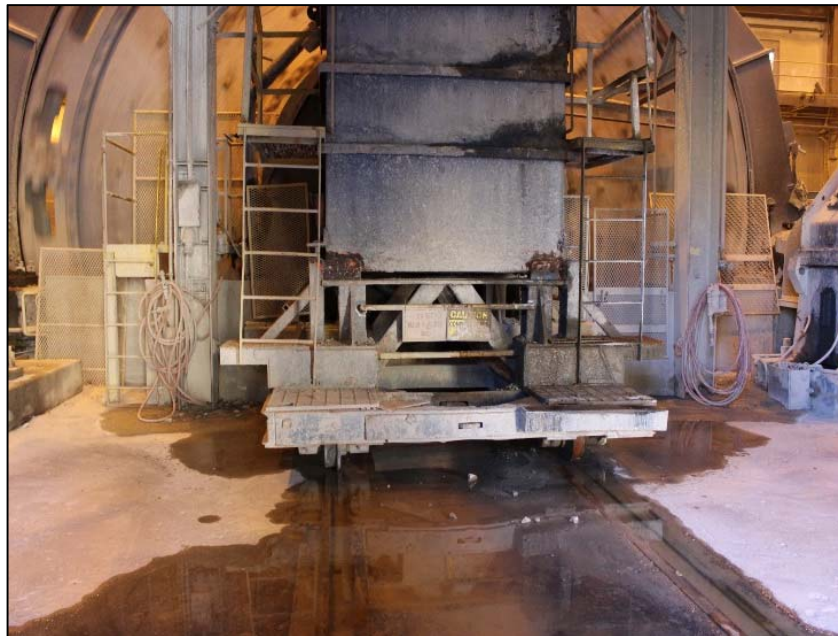
Existing Hazard(s) / Potential Consequence
