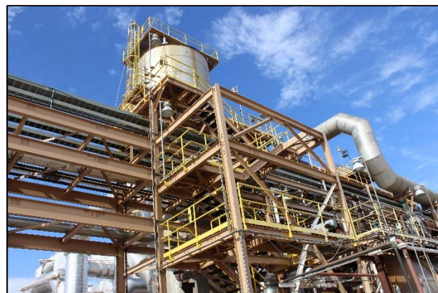
Fig 33 Railing systems and toe boards in place
