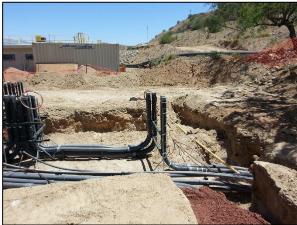
Figure 3.4 Trenching completed for electrical conduit installation; concrete-encased utilities showing red dye
