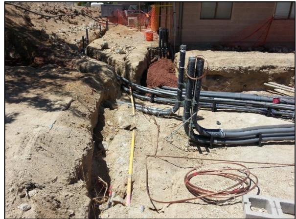
Figure 3.4 Trenching completed for electrical conduit installation; concrete-encased utilities showing red dye
