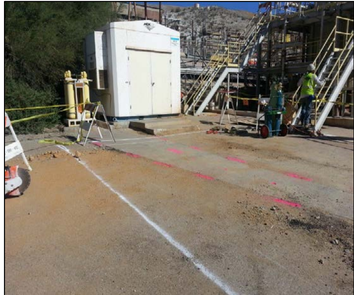
Figure 2.1 Perimeter marked with approved white spray paint
