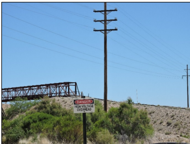
Figure 1.1 Look for hazards in all directions including up
