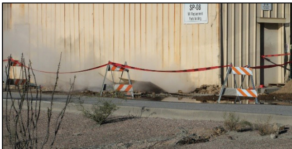
Fig. 1.4 Red flagging around a building
