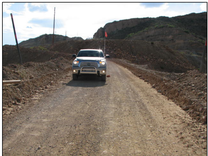
Fig. 2.11 Berms on a road
