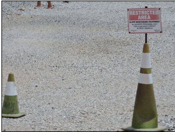
Fig. 2.2 Cones are used as a temporary barricade
