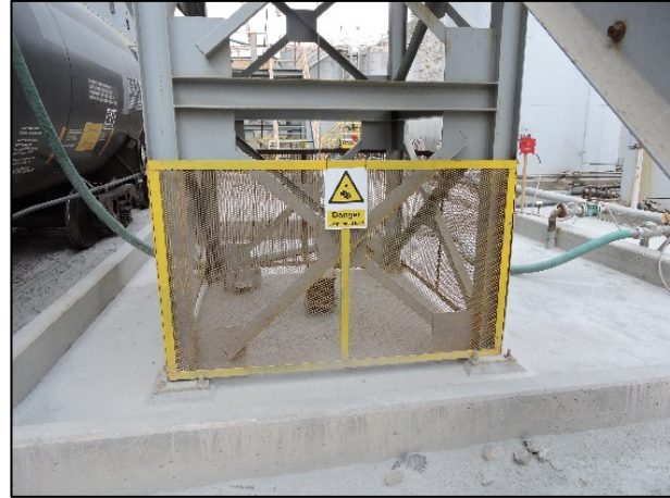
Fig. 2.3 Permanent barricade restricts access to a suspended load
