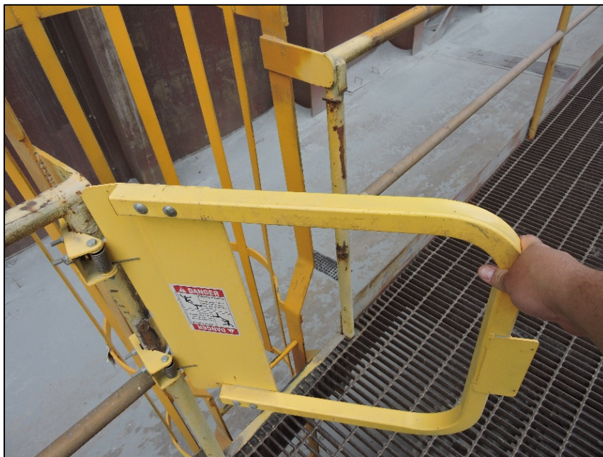
Fig. 2.6 Gates swing towards the employee when the transition is to a lower level
