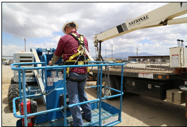
Fig. 30 Employee using Full Body Harness
