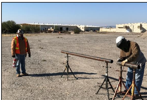
Figure 3.4 Fire Watch with fire extinguisher.
