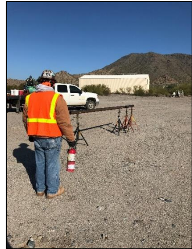
Figure 3.5 Fire Watch observing 60 minute wait period.
