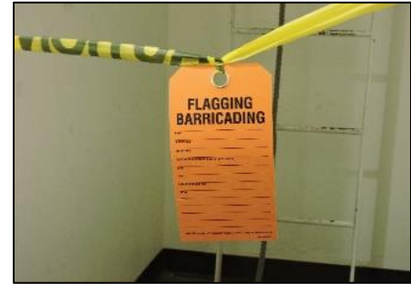
Figure 6.4 Flagging and tag used to warn others of possible hazard.
