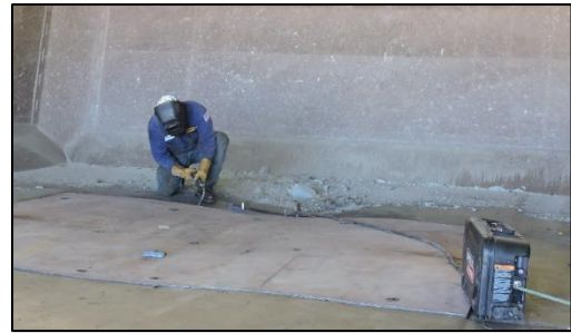
Figure. 2.1 Welder equipped with Nomex uniform, shaded lens, hood, and leather welding gloves.
