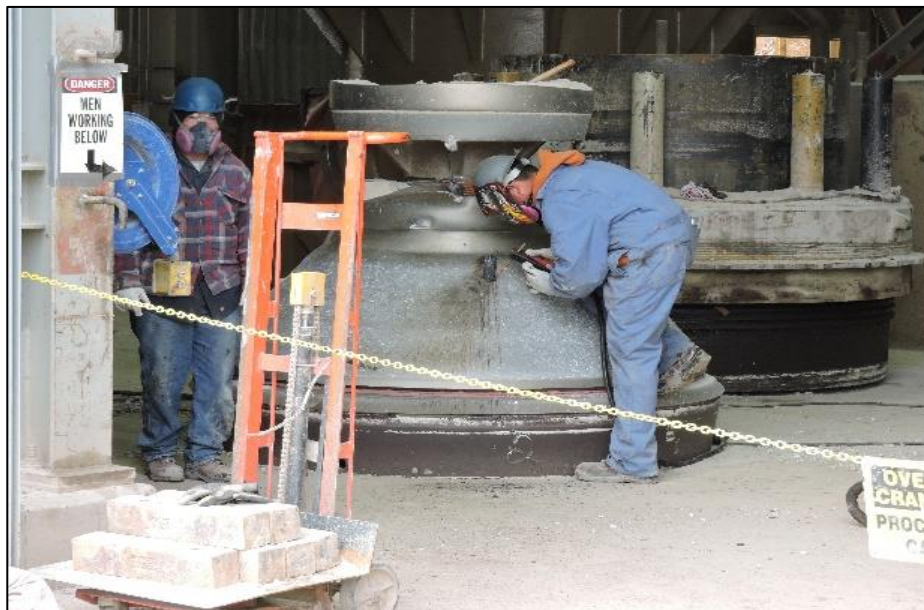
Figure 6.1 Fire Watch and PPE.
