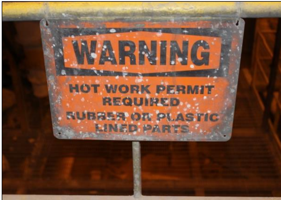
Figure 7.4 Signage warning of rubber or plastic parts in a High Hazard Area.
