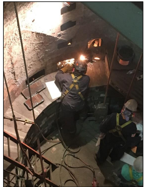
Figure 3.1 Hot Work being conducted by a Qualified Person.
