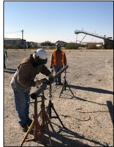
Figure 3.3 Fire Watch observing Hot Work.
