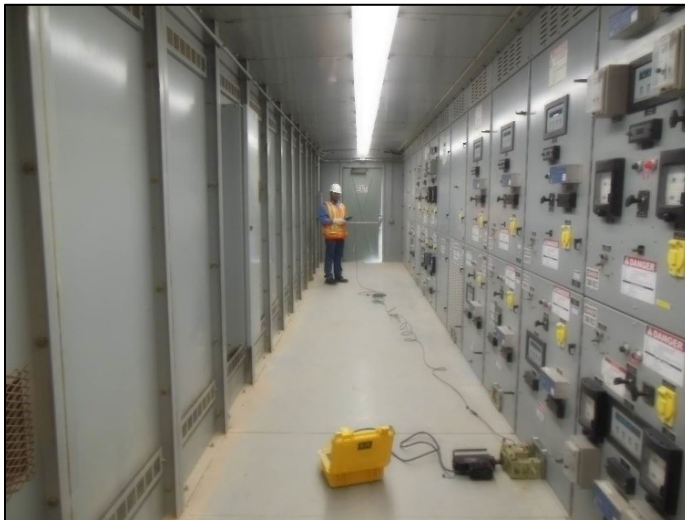
Fig. 2.22: Remote racking
