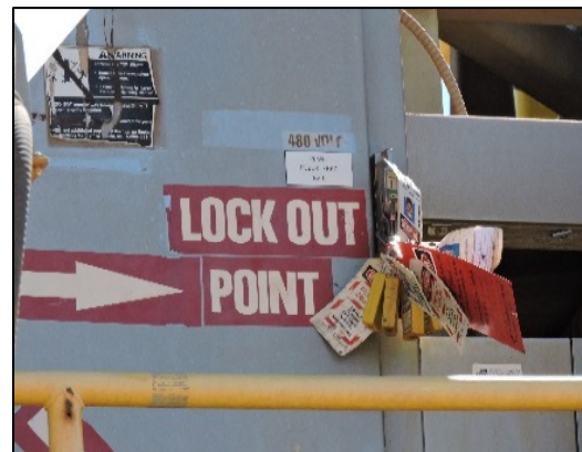
Fig. 4.7: A group lockout with multiple locks
