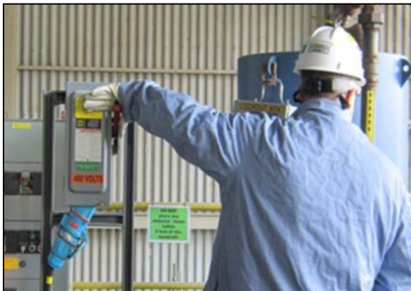
Fig. 2.30: Maintenance switch
