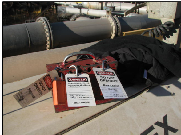
Fig. 4.8: An ECC lockout with multiple ECC keys and personal locks applied to a lockbox
