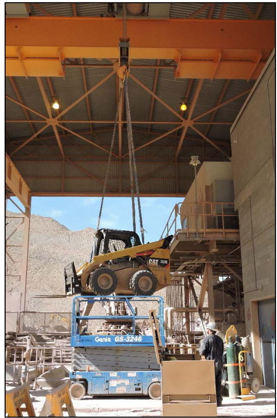
Fig. 3.1 Check travel paths when using lifting equipment.
