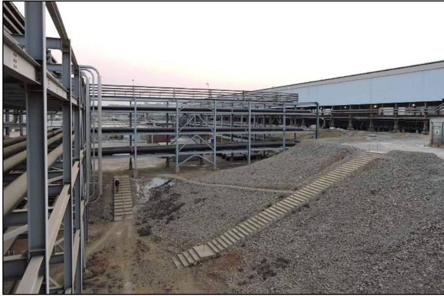
Fig. 2.7 Slope hazard mitigated with an engineering control (stairs).
