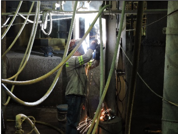
Fig. 3.2 Welding in a work area.
