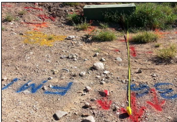
Fig. 3.32 Blue stake markings in a work area.
