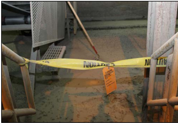
Fig. 3.31 Flagging and tagging in a work area.
