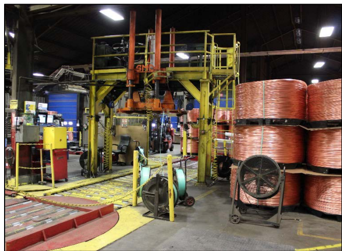
Fig. 2.4 Same work area from a closer vantage point.
