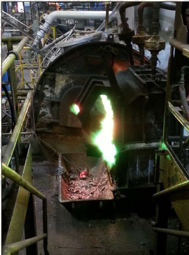
Fig. 4 Maintain an awareness of hazards while performing work.
