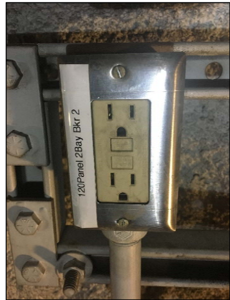
Fig. 2.8 Labeled GFCI outlet
