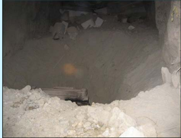
Fig. 1.6 View from outside of the ore pass
