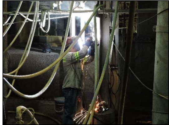
Fig. 2.15 Welding on the job
