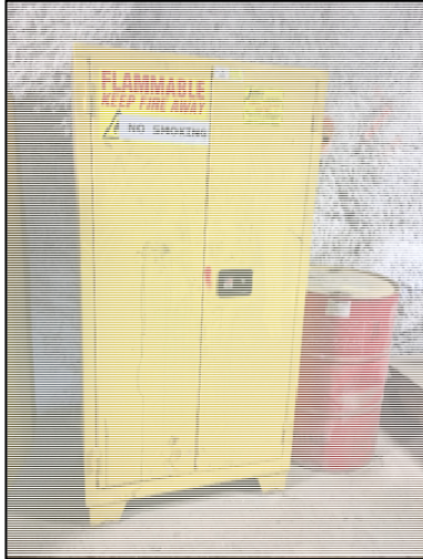
Fig. 4.1 Flammable storage cabinet
