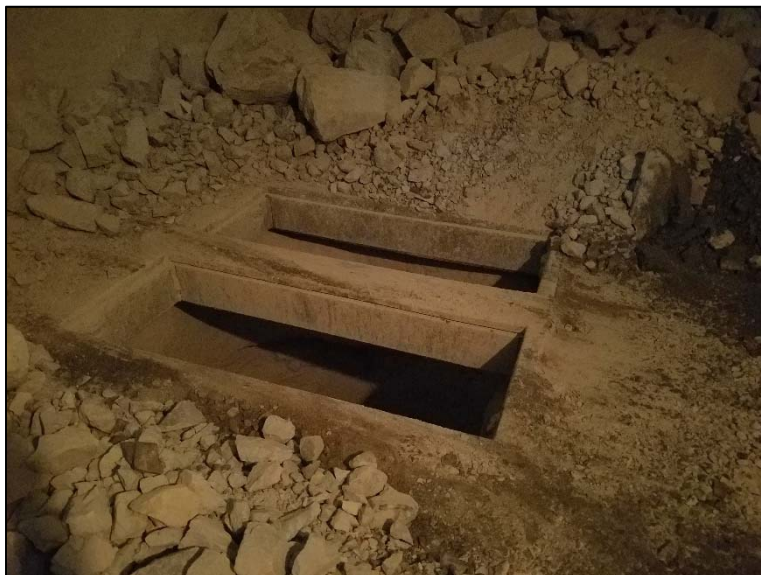
Fig. 2.32 Open holes pose a risk
