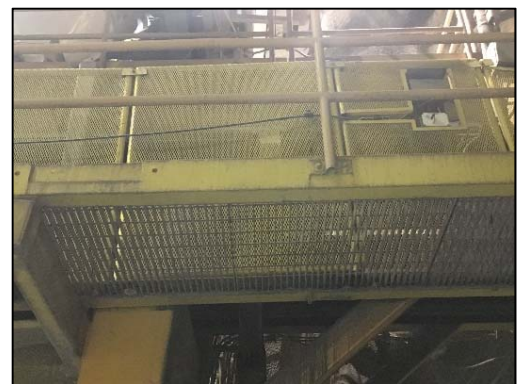
Fig. 2.28 Railing systems and toe boards in place
