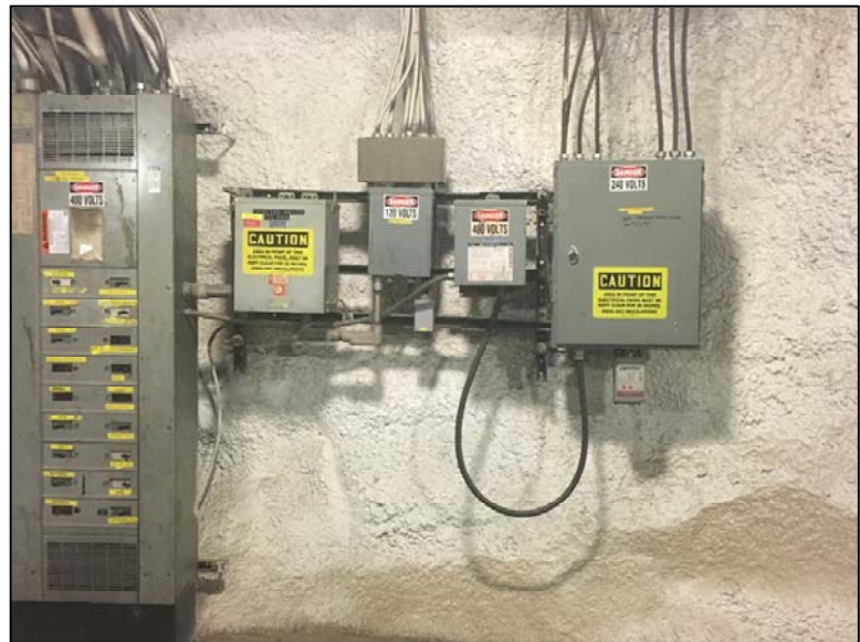
Figs. 2.6 and 2.7 Labeling on panels
