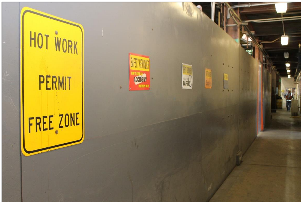
Figure 2.1: Signage in Hot Work Permit Free Zone
