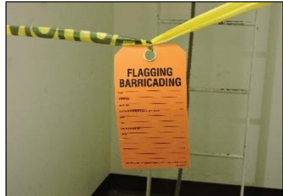
Figure 2.4: Flagging and tag used to warn others of possible hazard
