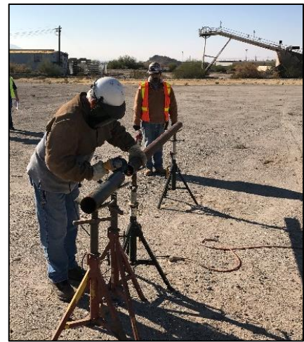
Figure 3.2: Fire Watch observing Hot Work
