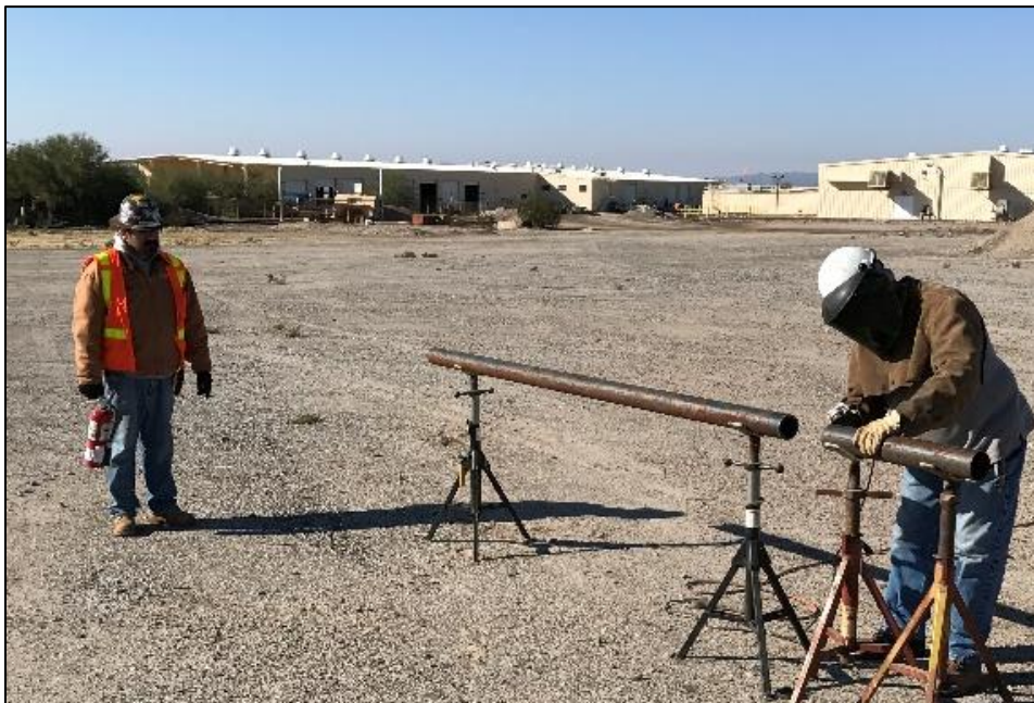
Figure 3.3: Fire Watch with a fire extinguisher
