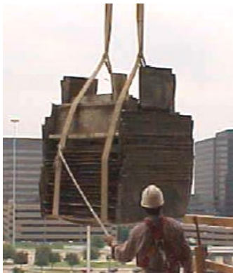
Figure 4.7: Choker Hitch
