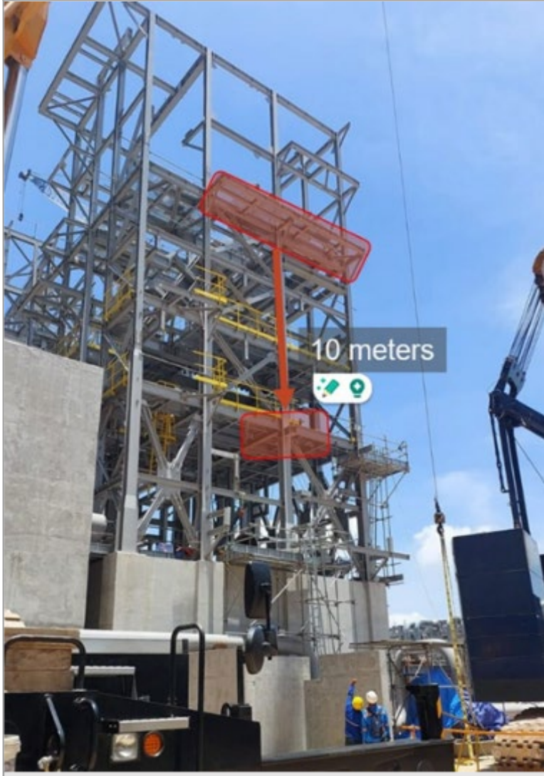
Scaffold grating weighing 20 kilograms fell 10 meters, striking an employee in a man basket.
