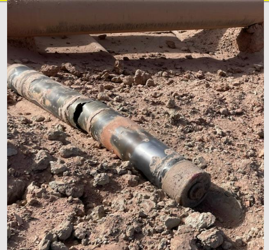
Worn idler that fell from conveyor
