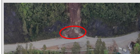
Small material retained inside the temporary berm.
