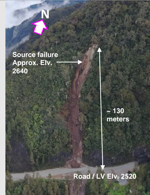
Source of the landslide came from upper slope. Consisted of topsoil, vegetation and boulders.
