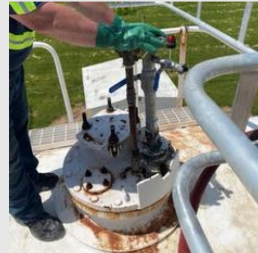
Re-enactment of valve assembly.
