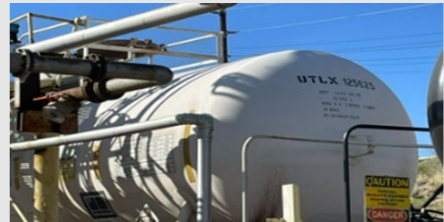
Work platform above the acid tanker car.
