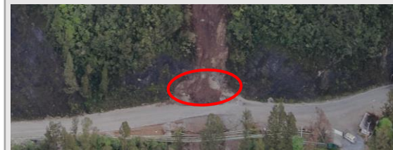
Small material retained inside the temporary berm.
