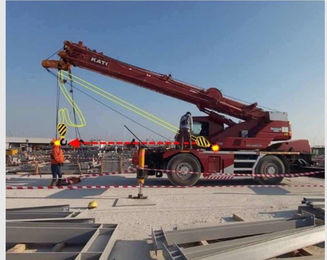
Illustration of crane hook movement when shackle broke
