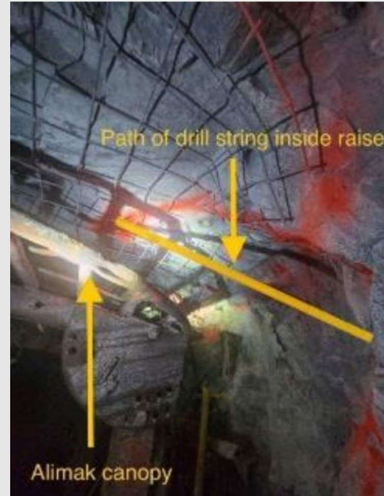
Photo from inside muck raise
