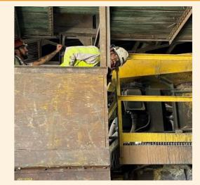
Dramatization of how the employee was pinned in between the railing and the crane cabin.
