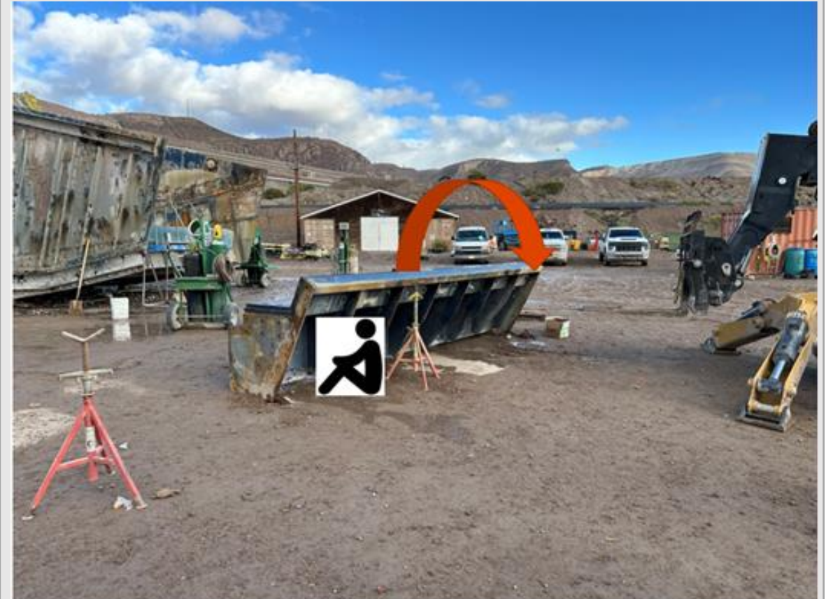
Position of employee, placement of pipe stands and direction the feed box tipped.
