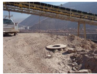
Missing or Inadequate Berm or Guardrail
