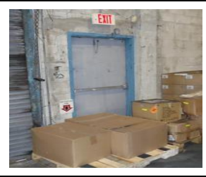
Damaged Emergency Lights/ Blocked Exits
