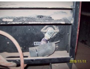
Unguarded Electrical Connections/Circuits
