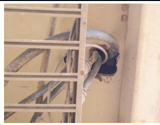
Improperly Bushed or protected electrical wires
