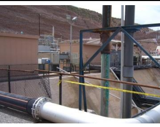
Damaged Hand railing, Toe Board, Work Platform
