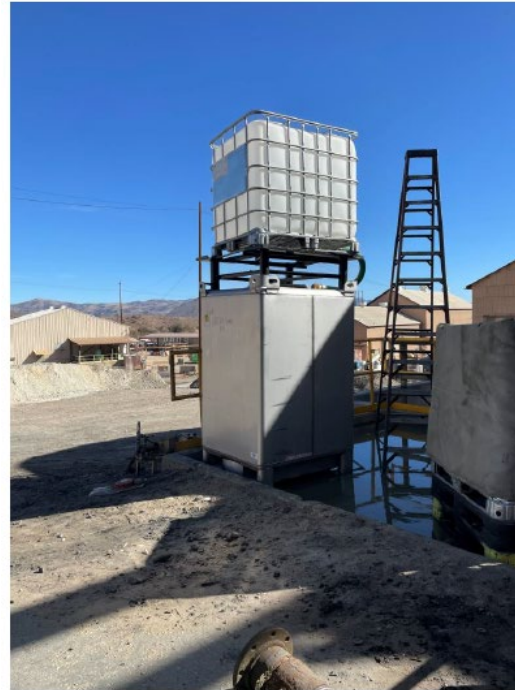
Tote- was empty- had rotated in frame in had been set on. Would not be stable in high wind determined by ease of shaking it. Need more diligence when set in holders or additional securement. D Bonilla arranged to stable-ize
