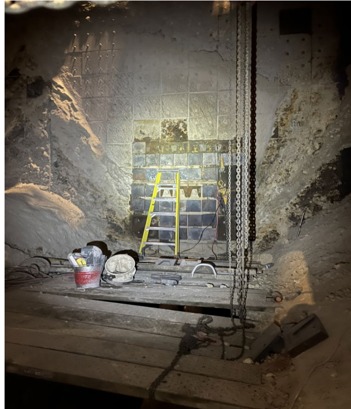
Liner event at Metcalf Mill Shutdown
