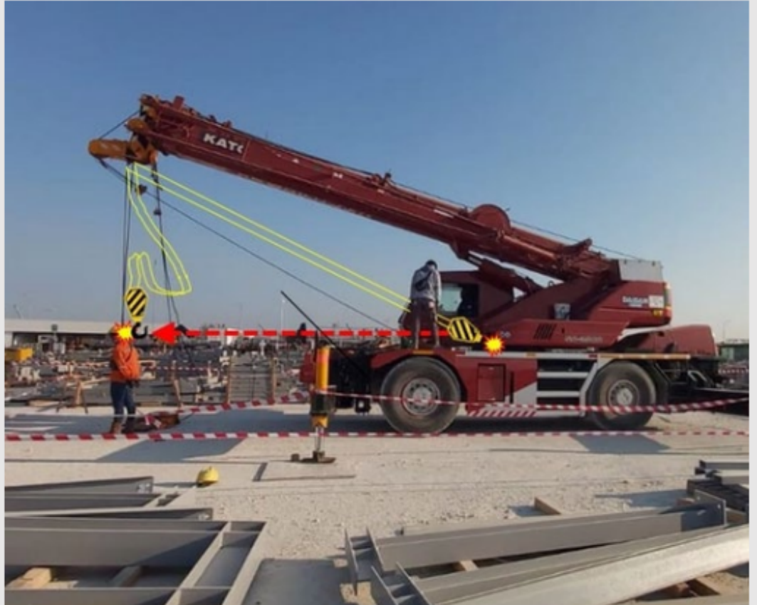
Illustration of crane hook movement when shackle broke
