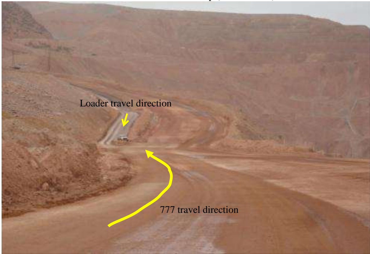
Base of the Northwest Ramp (LVA on Left)
