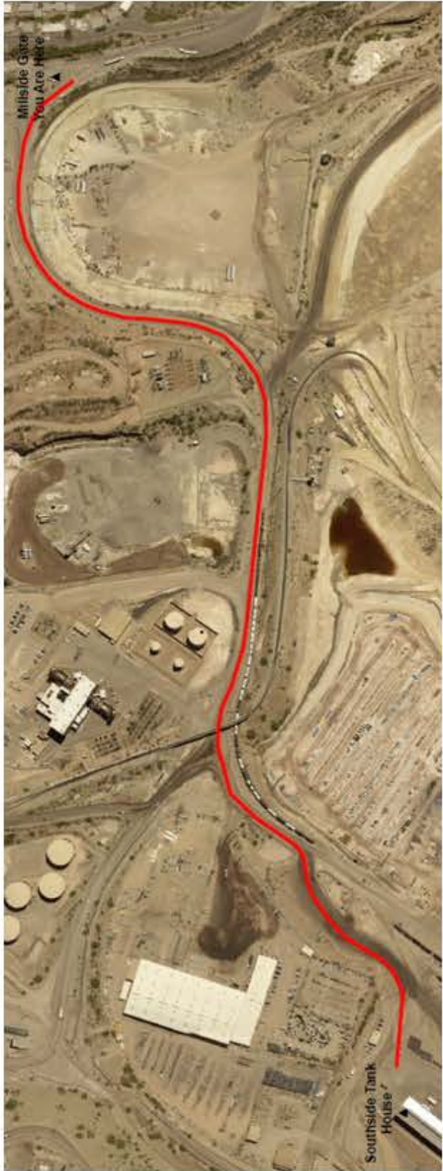
South Side Tank House
