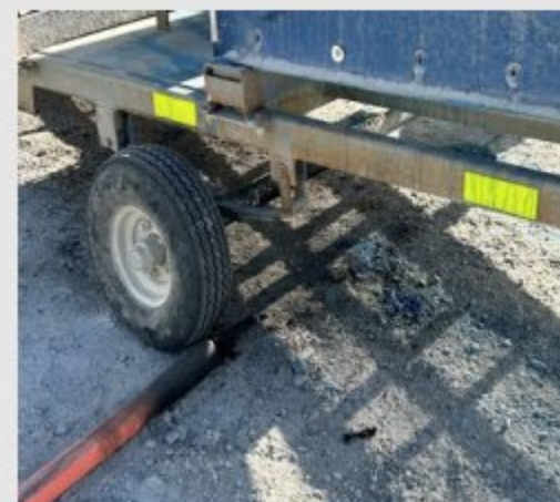
Broken cable following contact with portable restroom trailer.
