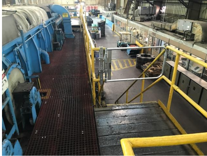
Newly Installed Stair Landing Gate
