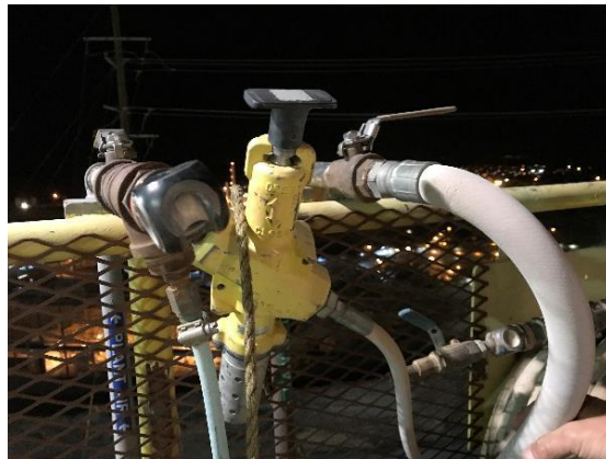
Photo 5 Norgren In-line Lockout Valve - Plunger Knob on top / bleed off on bottom
