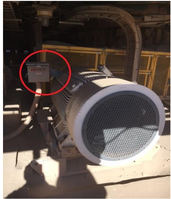
Mounting location for motor tap box
