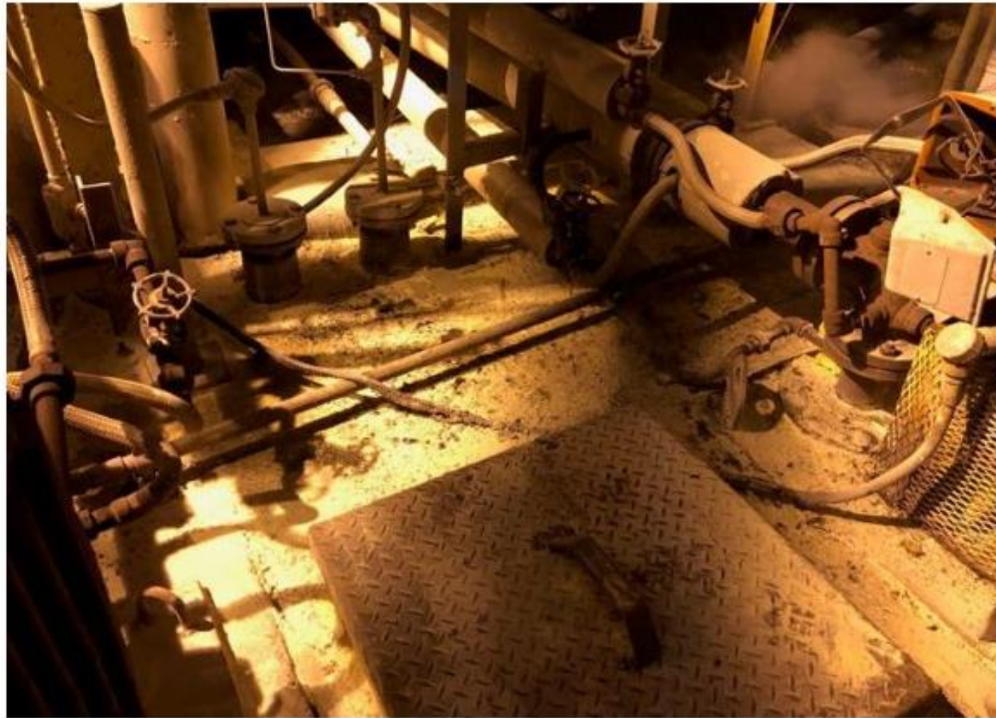
Burned power cables to the sulfur pumps.
